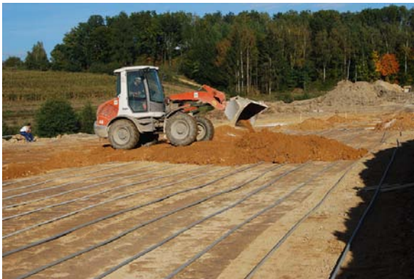
Figure 1: Installation of a horizontal heat collector system near Viechtach (Bavaria/Germany).
